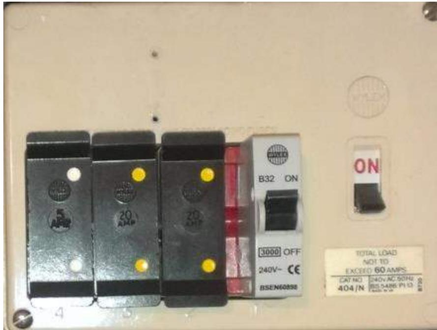
**HOWEVER** many of these then do not allow the fuse cover to be fitted back on, leaving gaps where the live terminals are (some boards have bigger gaps than other with the fuse cover removed). Not only should the correct **type** be fitted, but the correct **rating** for the circuit type (and cable sizes, etc) too, or you will add more problems, rather than solve them!
