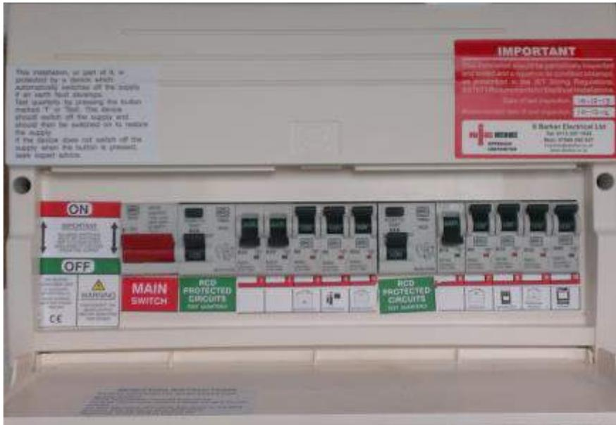
2 RCDS fitted, each controlling several circuits
