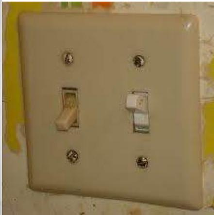
There should be no metal fittings if these older fitting are in use, as this is almost certain to still have original wiring, which is not likely to be earthed. If ALL fitting are plastic (or ceramic/Bakelite) then this is not an issue.
