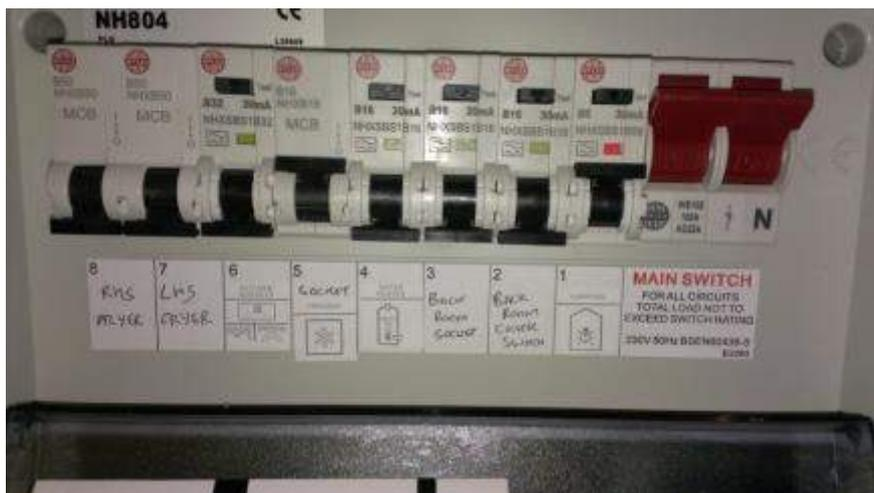
Individual RCBOs fitted (with the little black test button – usually yellow!) so each circuit has it's own individual RCD protection – Perfect for minimising disruption to other circuits on Commercial and Industrial Installations.
